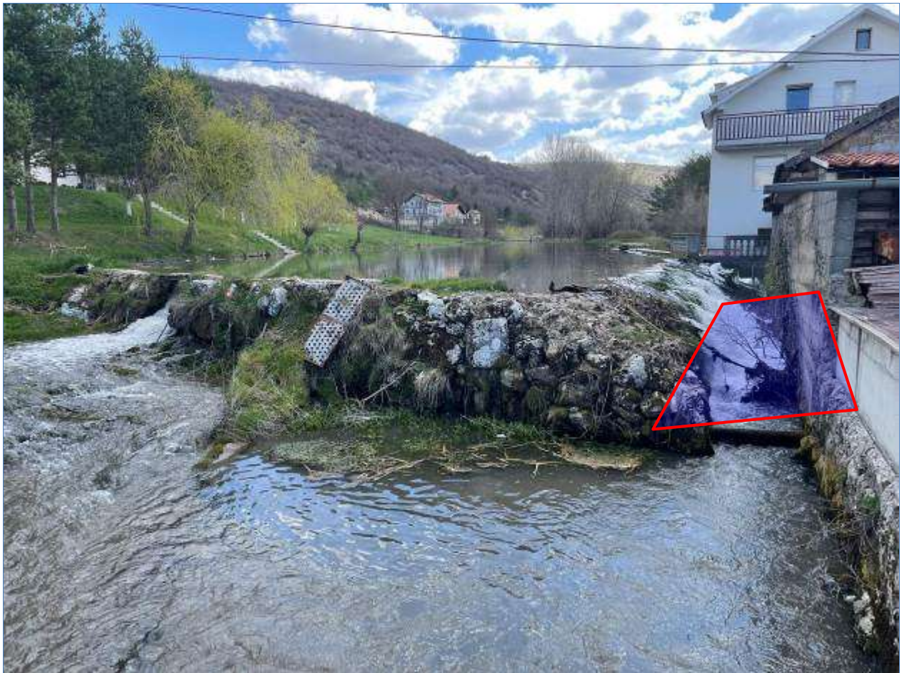
Figure 24. The spatial position of the channel used to direct water onto the mill blades..
