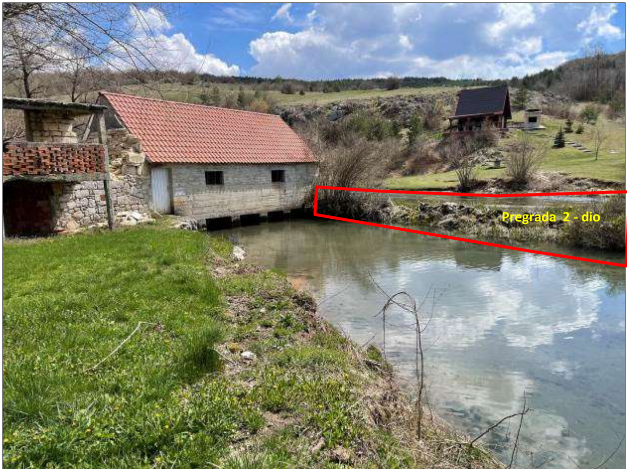
Figure 30. The part of the canal downstream from Kelavin's Mill with the initial section of the second barrier planned for removal
