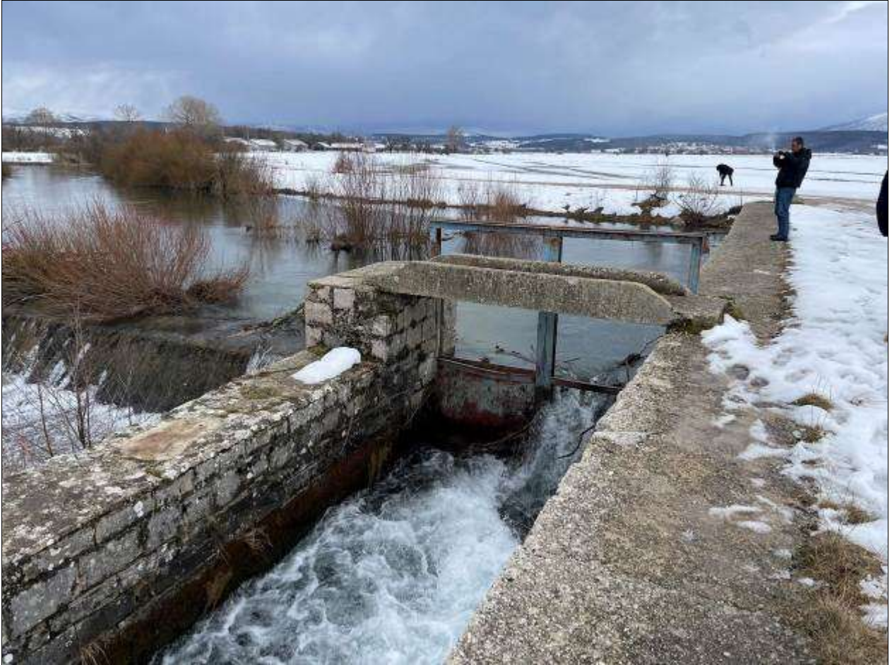
Picture 9. The weir along the left bank of the riverbed no longer serves any hydrological function and therefore requires removal
