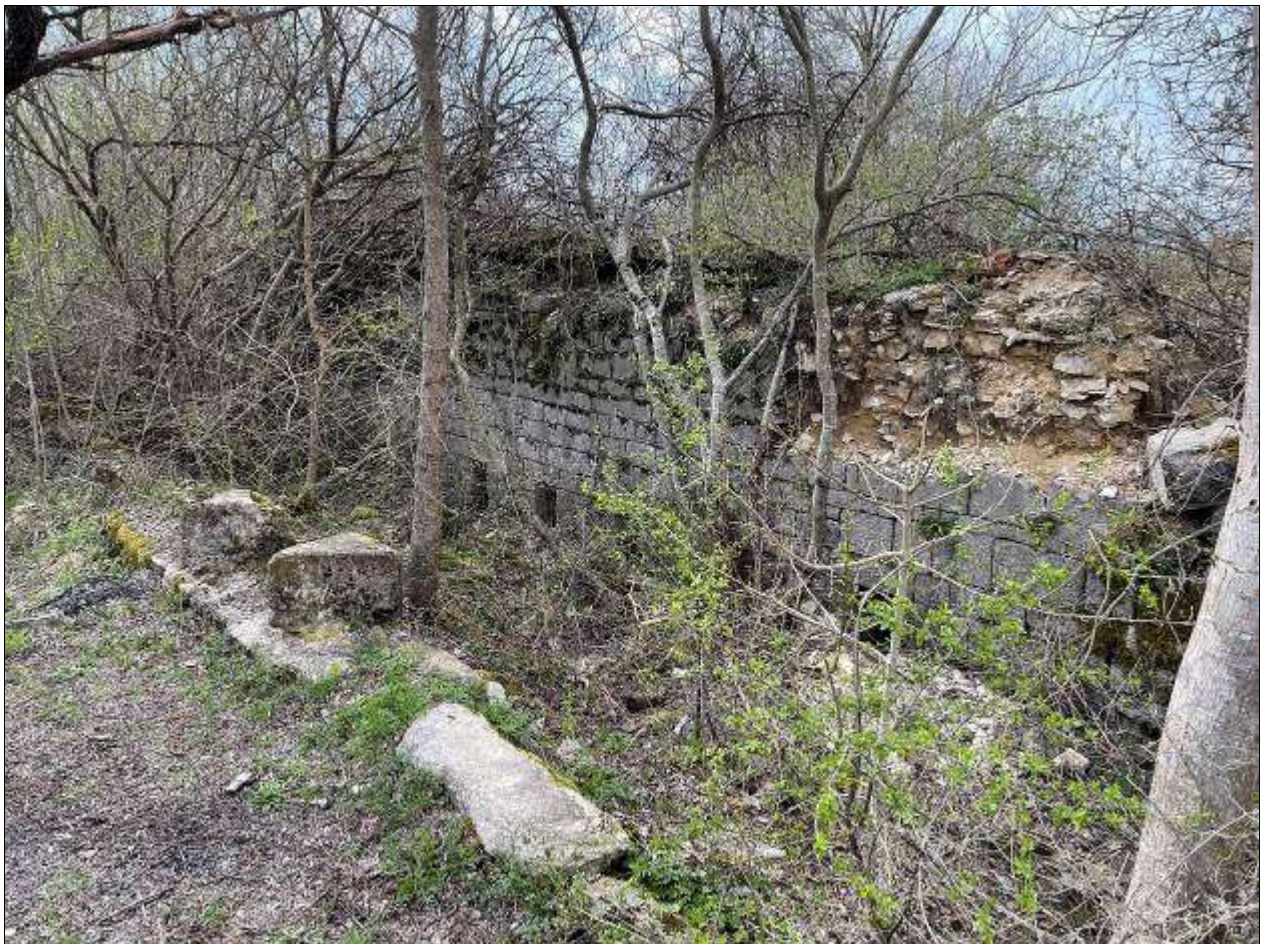
Figure 34 The ruins of the former building (mill) with stone weirs used to direct water to the wooden turbines of the mills.
