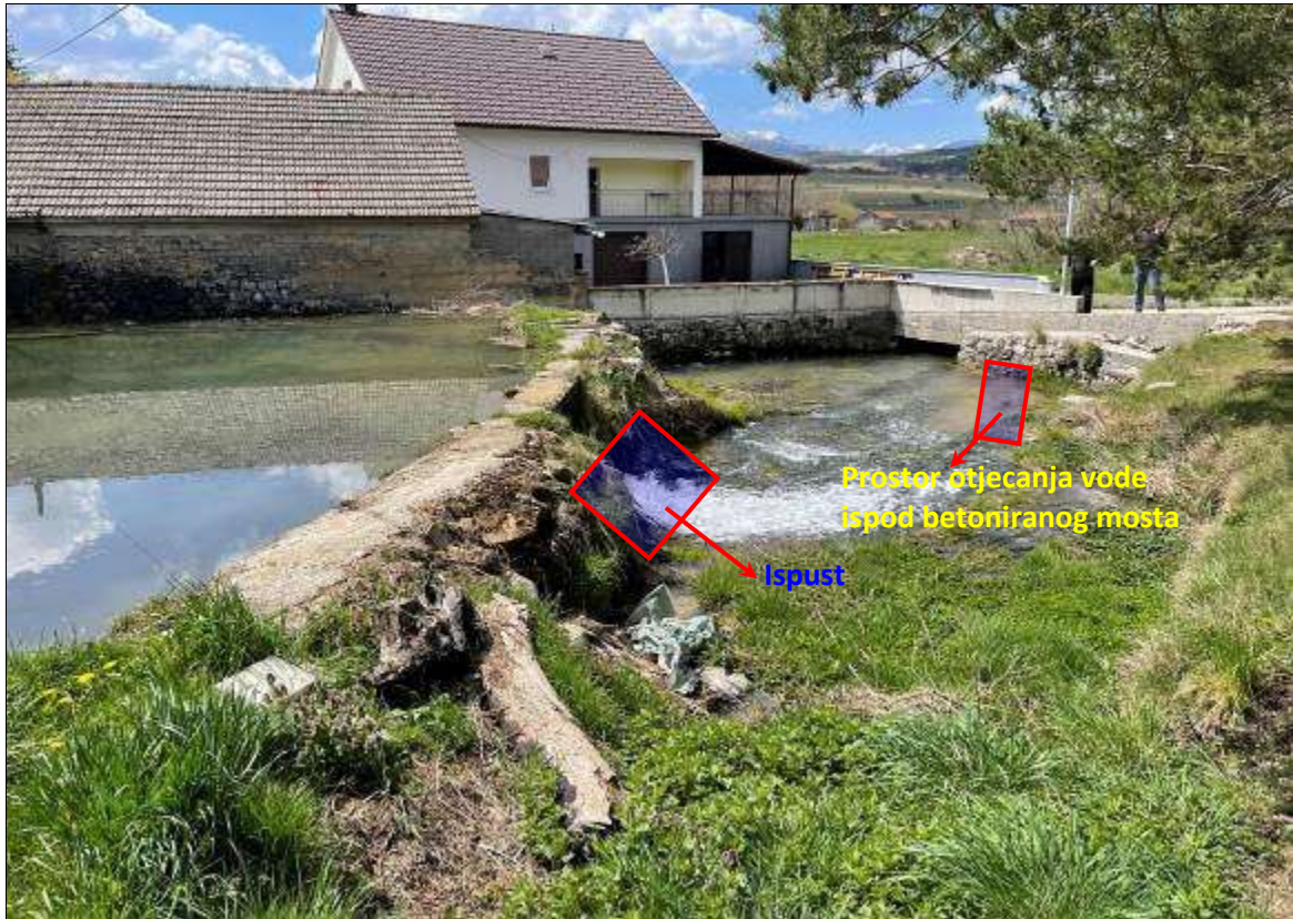
Picture 22. Spatial position of the transverse barrier with the position of the overflow opening for the discharge of excess water accumulated in the dammed area.
