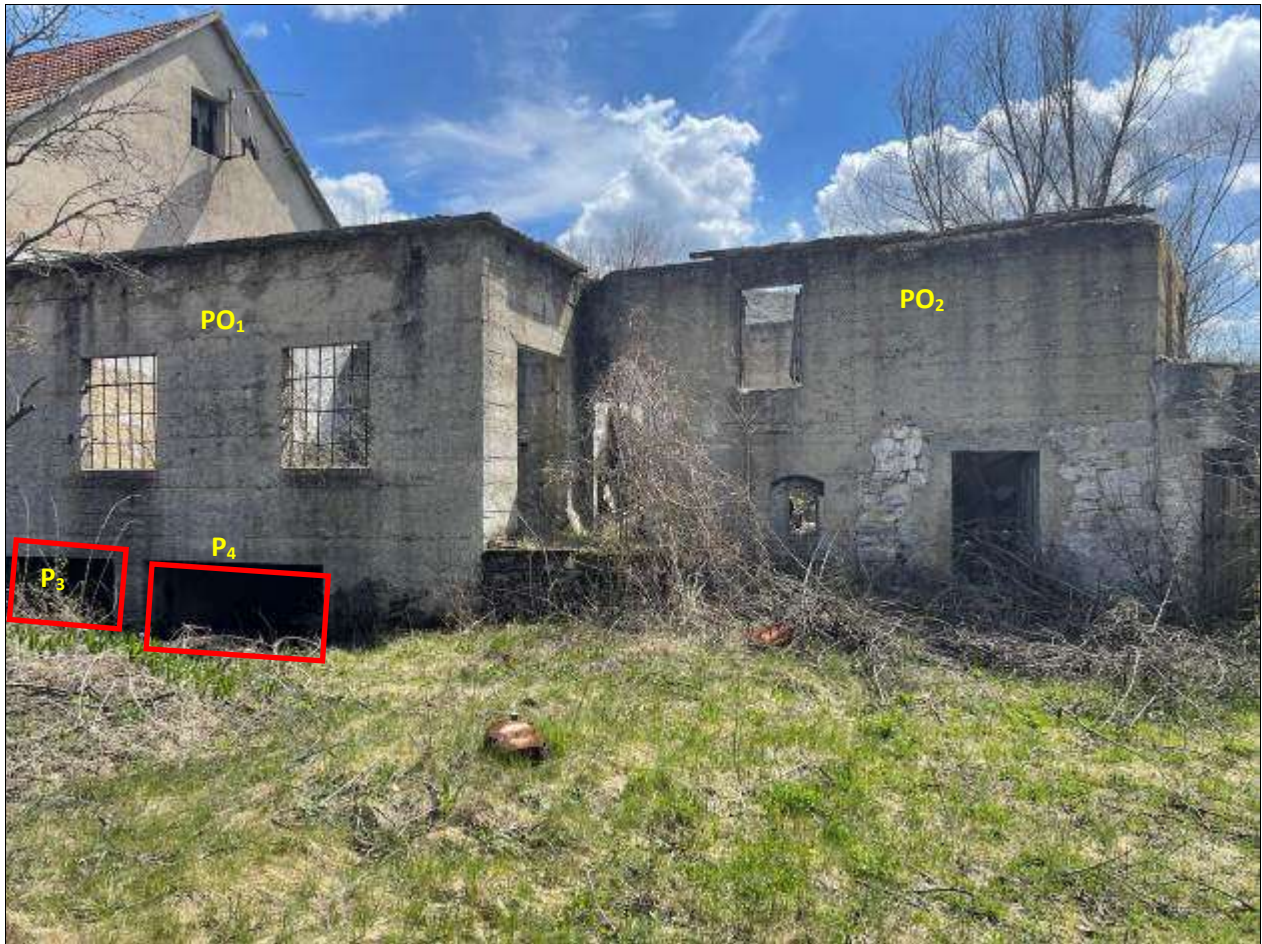
Picture 16. Spatial position of the unreconstructed objects that obstruct the right branch of the Sturba River in the area of Mljekara Orman
